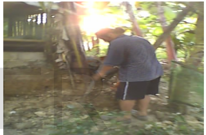
Plate 2. Leveling of Soil
